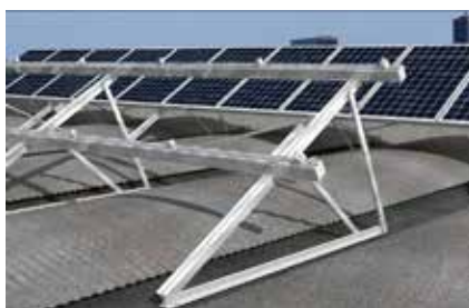
Flat surface PV installation
